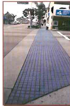
Cast-in-place sidewalk and cross-walk materials, such as concrete, can be textured and colored to define pedestrian areas on the parkway.
